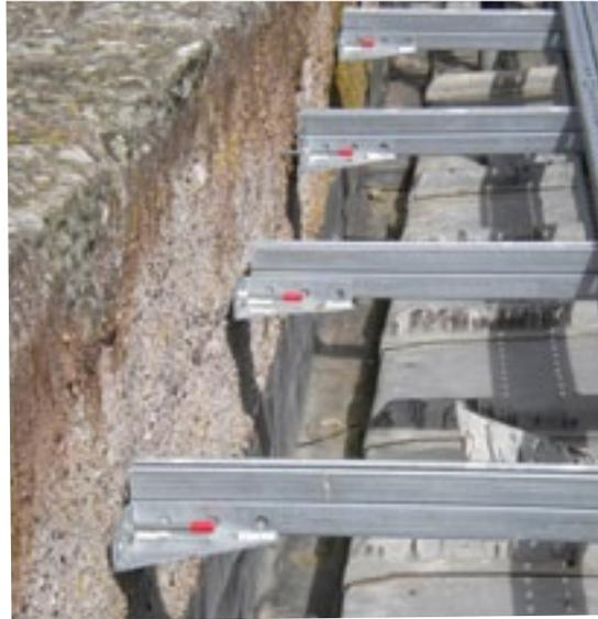
The design utilises a light weight 'uni-strut', hot dipped, galvanised frame system which will minimise the load on the castle walls. The galvanised system will suit the potentially corrosive environment at the castle. Bespoke wall brackets were also designed to minimise weight load issues.
