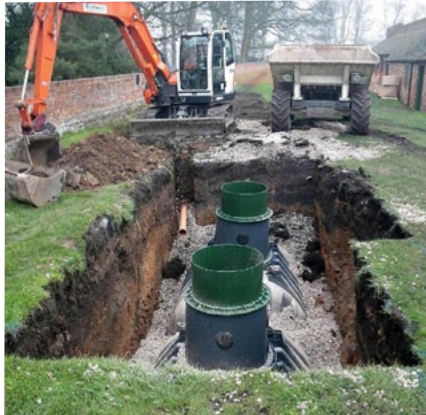
Left The only visible parts will be the manhole covers, underneath which the filter and pump can be inspected
