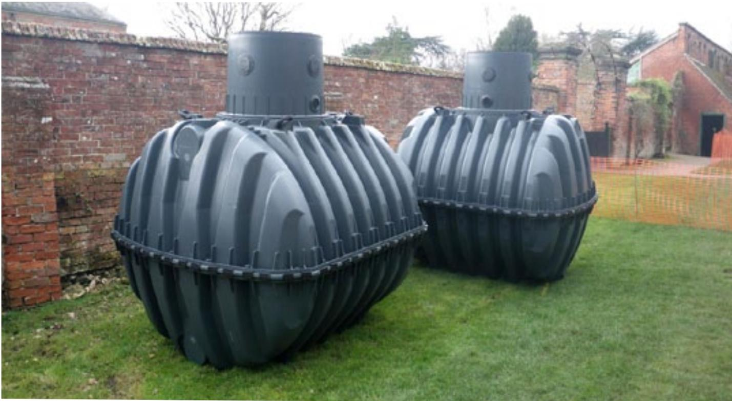
Top left **The image shows the grey turret on each tank in which the leaf filter is mounted. Rainwater flows in through a four inch pipe; the filter diverts clean water into the tank**
