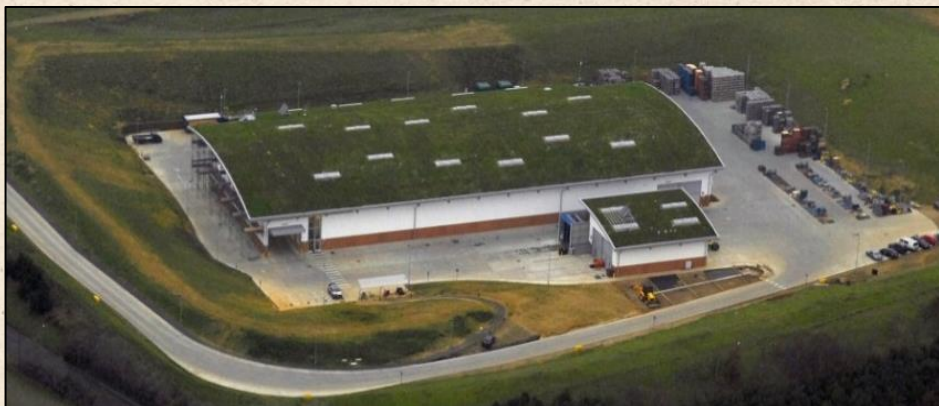
Adnams Eco-Distribution Centre
